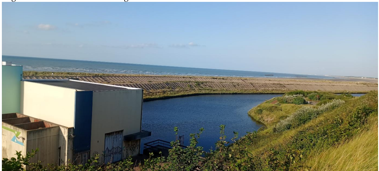
Figure 8. Alliés dike near the Texier pumping station (Field survey, Diouf, 2025).
