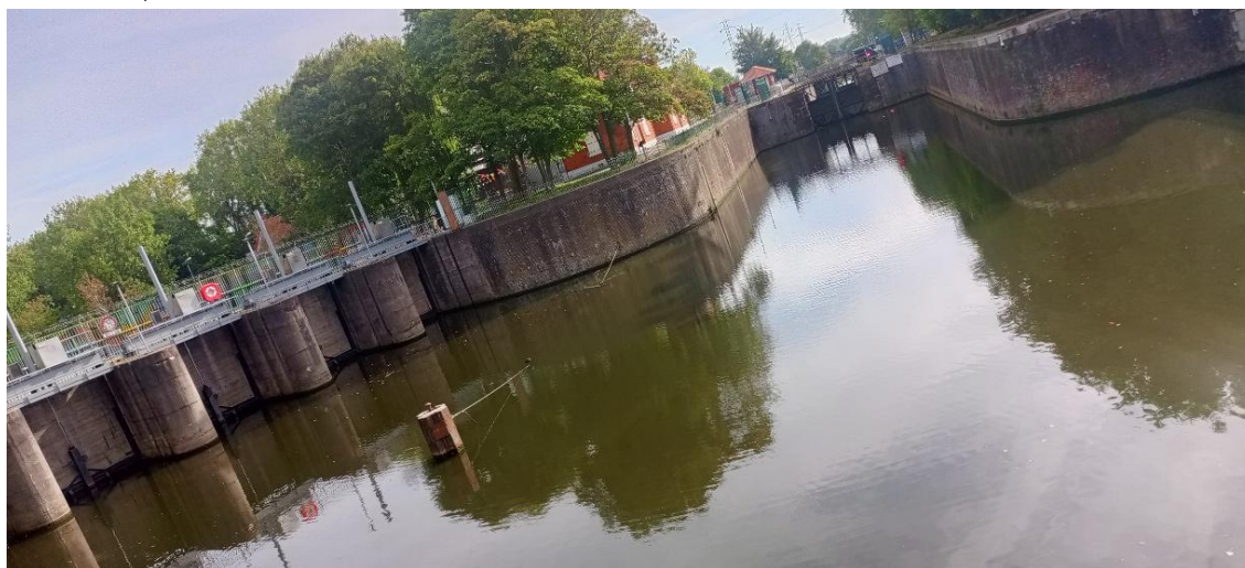
Figure 2. Location of the four locks in the Dunkirk area (Field survey, Diouf, 2025).
