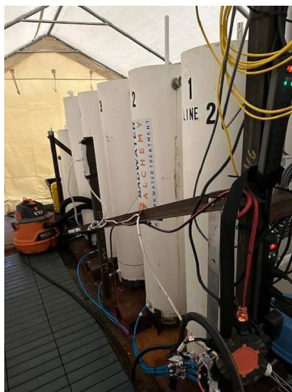
Figure 2. The Generation 1 pilot system looking down the row of reactors in Line 2 showing the air manifold and delivery lines. All processing is controlled via a PLC.
