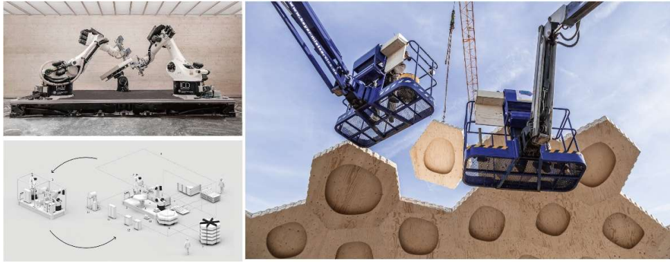
Figure 3. Pre-assembly timber structure (left) and the on-site assembly of large components (right) © University of Stuttgart [16].
