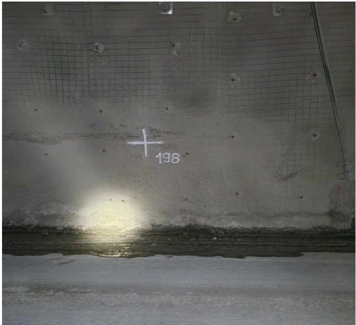
Figure 6. The ground control mark used in the underground mine.
