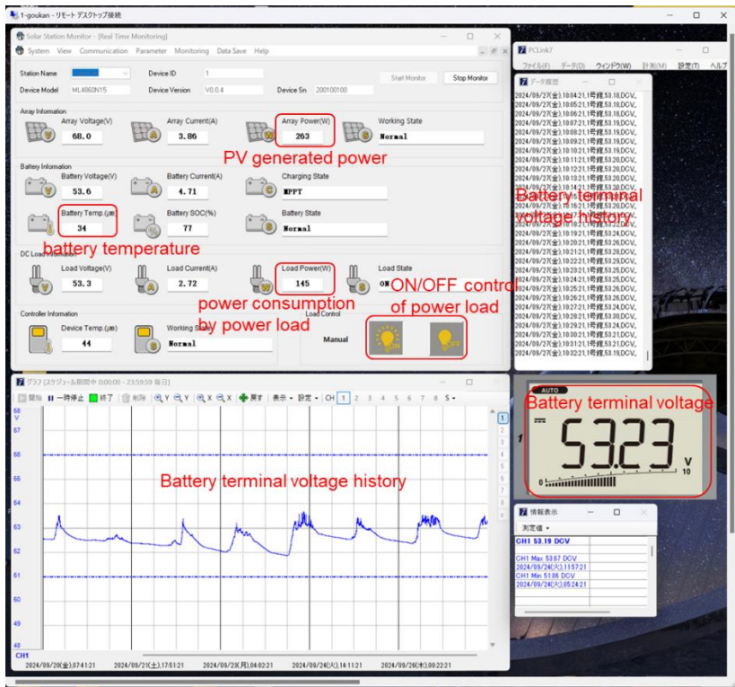
Figure 7. Monitor screen of the microgrid operation.
