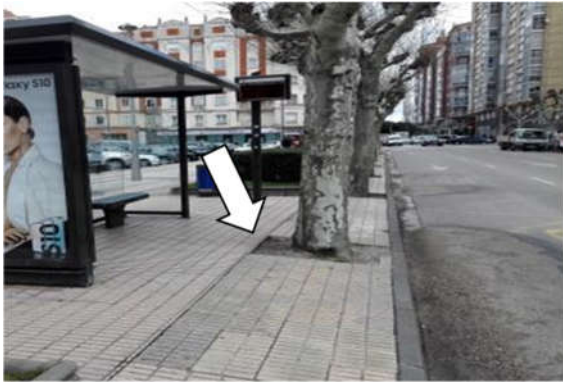
Figure 13. Tree pits not flush with the pavement.
