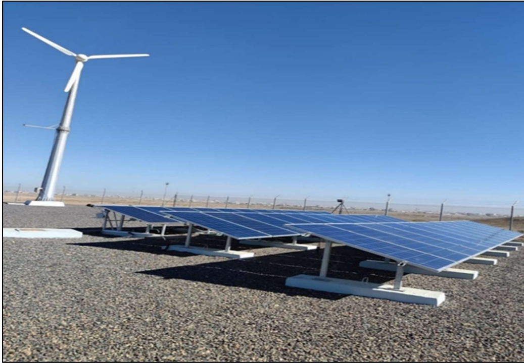
Figure 36. REEEC operates solar systems with an overall capacity of 9 kilowatts. Electrical characteristics are provided under standard test conditions (STC) with an irradiation of 1000\text{W/m}^2 , a range of 1.5 air mass, and a cell temperature of 25^\circ\text{C} .
