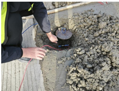
Figure 3. Temperature and humidity sensors.
