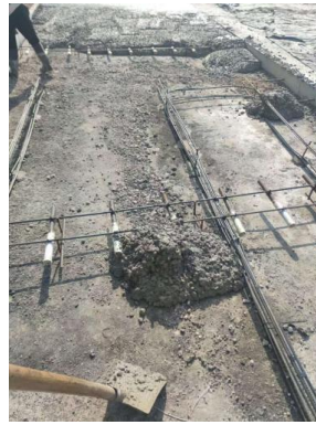
Figure 4. Strain and stress sensors.
