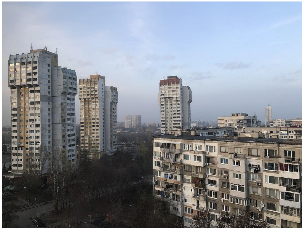
Figure 16 Apartment blocks in Sveta Troitsa, Sofia, Bulgaria, at the northwest end of the district, next to a train station [59].
