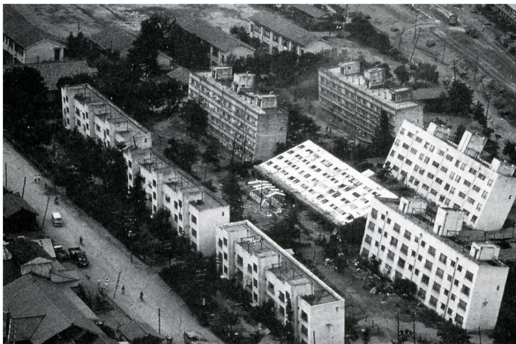
Figure 9. Rotations of four-story residential apartment buildings at Kawagishi-cho, Niigata in 1964 (Photo, USGS Archive).
