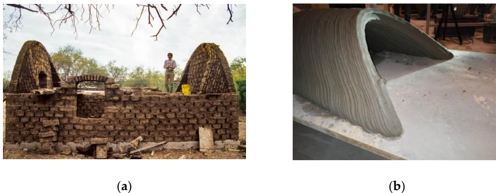
Figure 4. the Nubian vault: (a) Traditional Nubian vault construction technique using raw earth bricks [21]; (b) Prototype of a vault 3D-printed with 40° inclined layers without supports [22].
