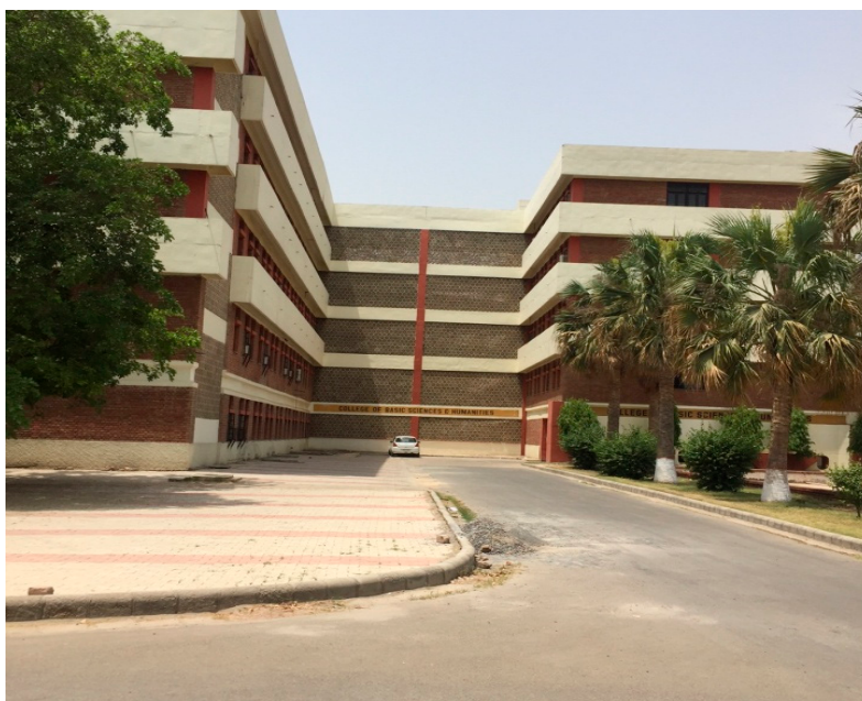
Figure 1. Multi-storey building of the College of Basic Sciences and Humanities where Apis dorsata made nests at different ceiling projections of the building (Adapted from Sihag 2017).
