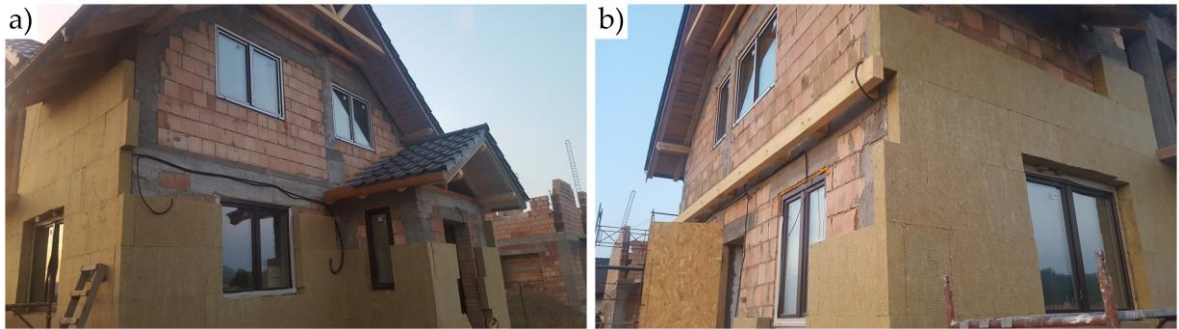
Figure 5. Photographs of the mineral wool insulation of the case study building during the construction stage, in 2019
