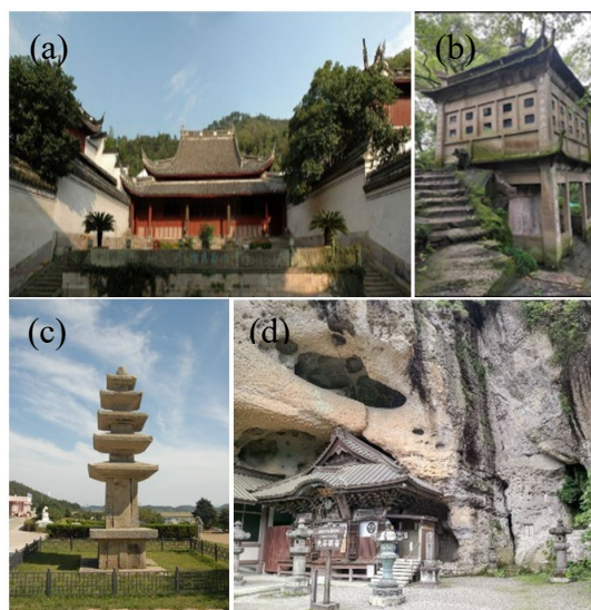
Figure 4. Examples of tuff-built AHS in East Asia: (a) Baoguo Temple, Ningbo, China, (880-1013) [28], (b) Sanlao Stone House, Zhejiang, China (1921) [30], (c) Korean Treasure 529, Jingdo, S.Korea (918-1392 CE) [31], and (d) Oya-ji Temple, Kanto, Japan (810 CE) [32].
