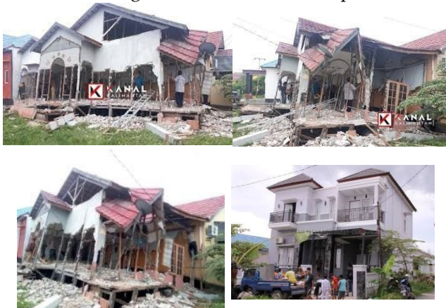
Figure 13. House Building's collapsed.
