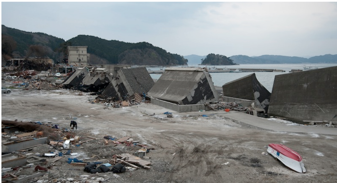
Figure 1. Pieces of the Tōhoku multi-billion dollar tsunami protection wall after a level-2 tsunami hit the coasts of Japan in 2011. While each individual concrete section of the wall did not suffer significant damage, the erosion at the foundations of the wall happened so quickly that the concrete barrier simply fell (Picture from [1].)
