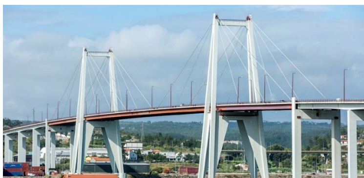
Figure 1. General view of the Edgar Cardoso Bridge in Figueira da Foz.
