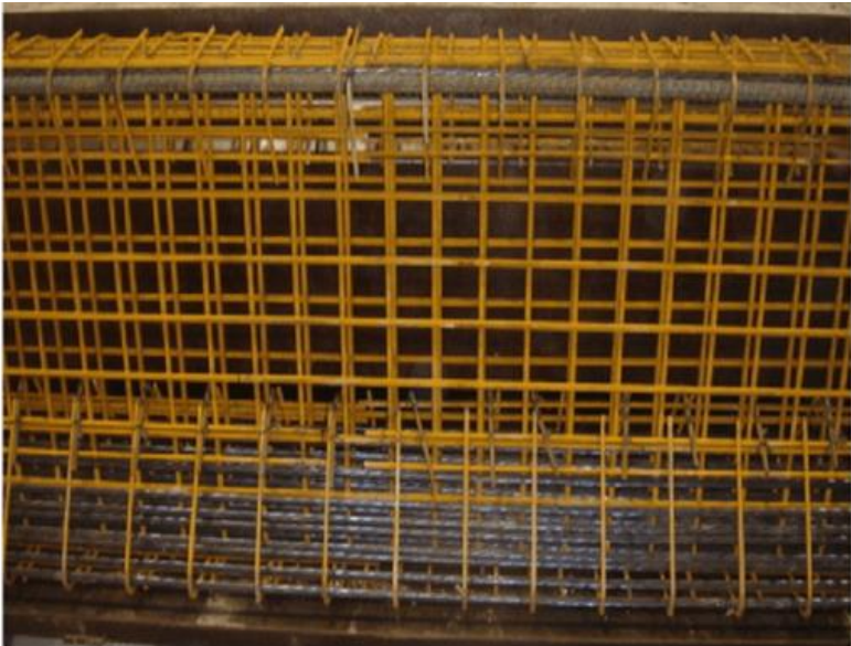
Figure 4. I-girder heavy reinforcement (poured with fly ash concrete) [69]
