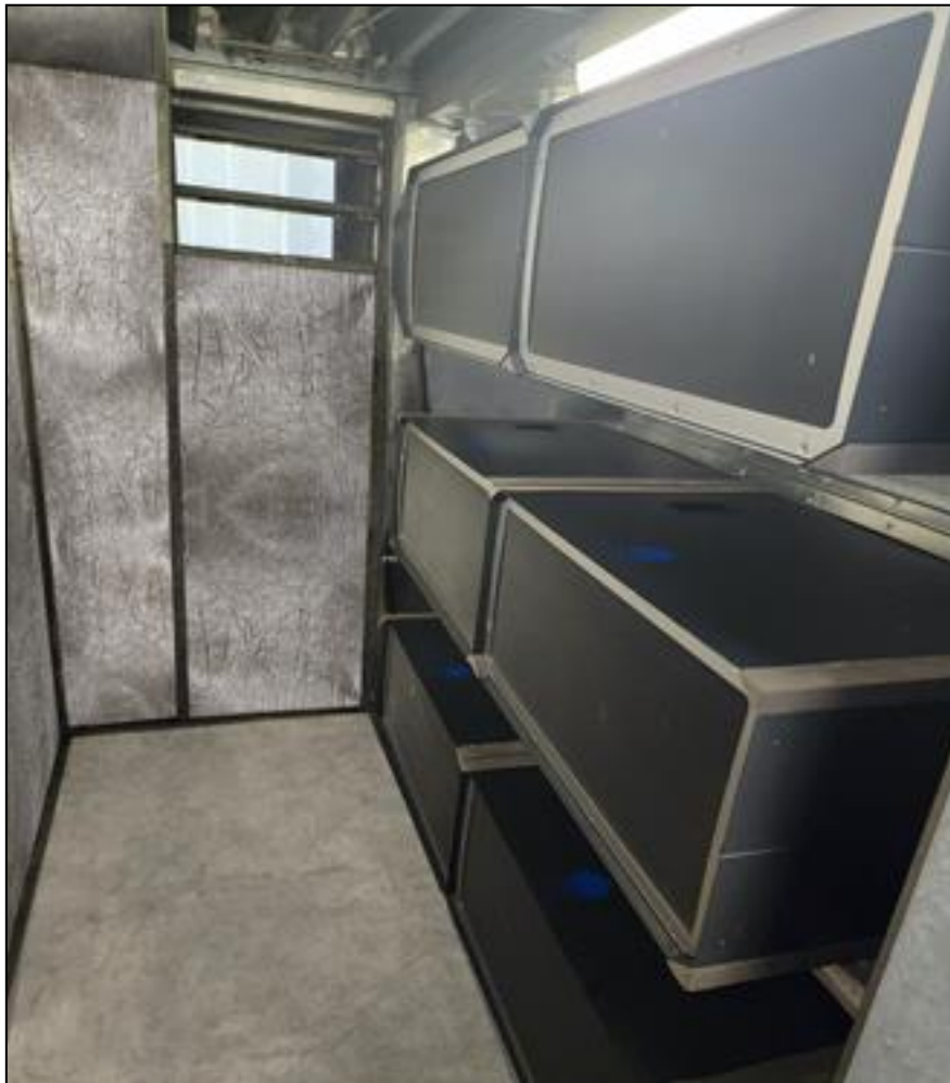
Figure 2. Six PlasmaShield units located in the air handling unit.
