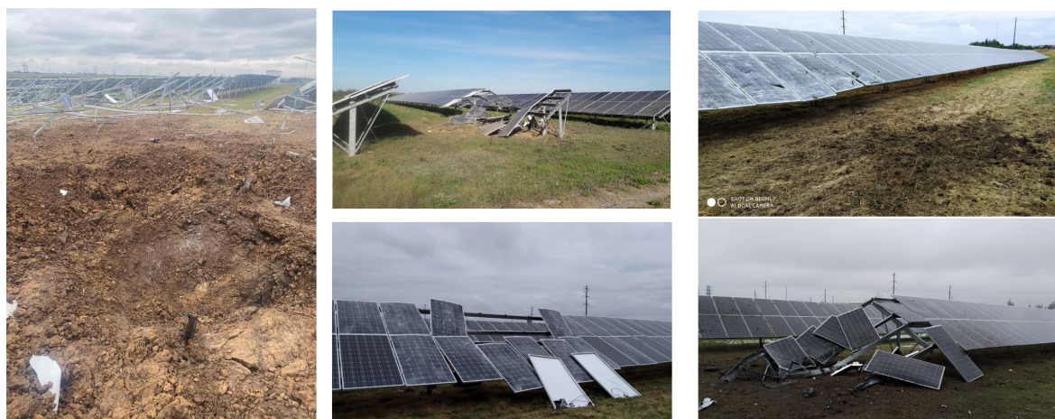
Figure 2. Damage to the photovoltaic modules at the solar power plant as a result of missile strike
