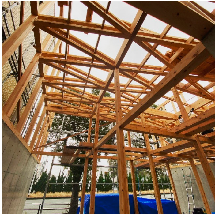
Figure 6. Erection of superimposed open-work girders (Authors).
