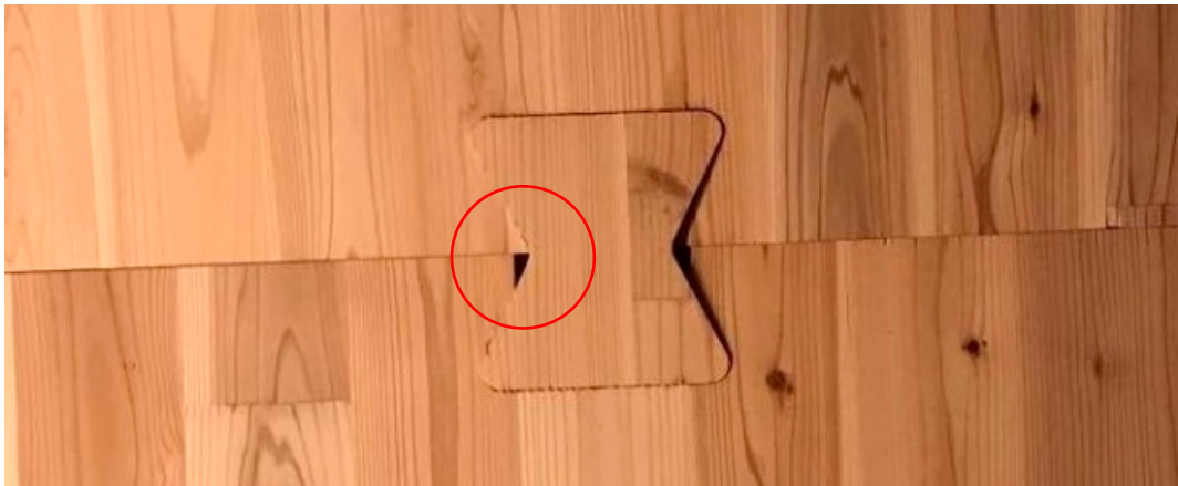
Figure 15. Localized Lamina Chipping at Connector Key Insertion (Authors).
