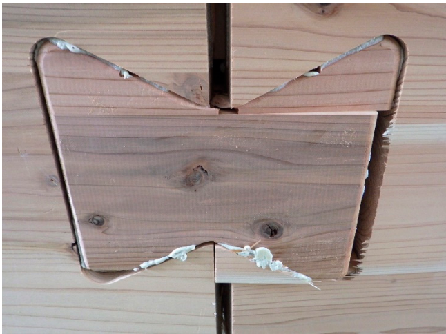
Shear failure for snagging
