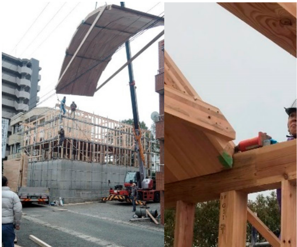
Figure 23. Erection and Alignment of CLT Arch Modules (Authors).
