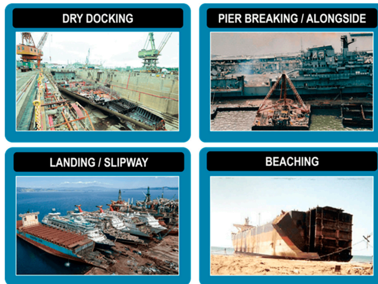
Figure 1. Ship Recycling Methods.
