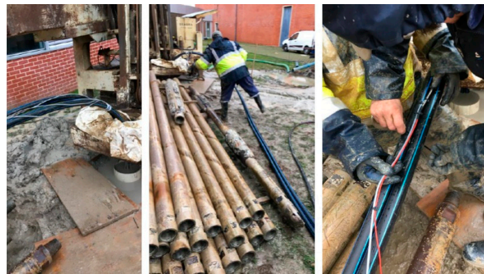
Figure 6. Installation of the temperature probes for the monitoring system.
