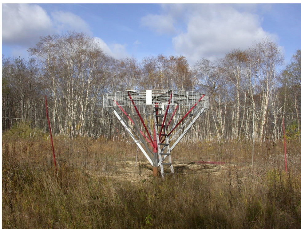
Figure 1. Installation of the Pole-2 instrument at the observatory.
