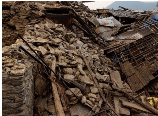
5 (c) Full collapse of the short wall
