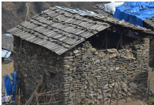
5 (a) Out-of-plane structural loss of end wall
