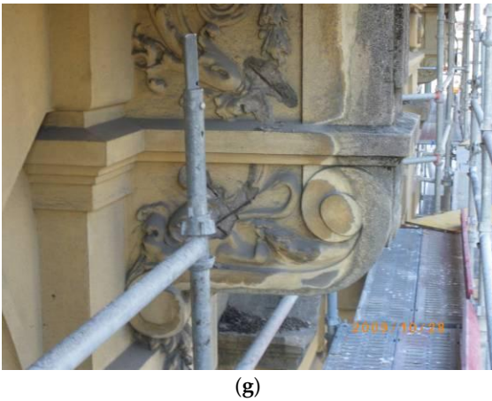
Figure 2. Sampling performed on facades of TNSJ. Samples: a), b) FPo-2 Polymorphic motif (Zone evidently subjected to recent intervention, sample drawn by hand); c) FPo-8 Mask; d) FPo-10 Geometric ornament; e) FPri-A1P1 Frieze; f) FPri-PB Frieze, bottom part; g) FN-V2P1 Flower ornament.
