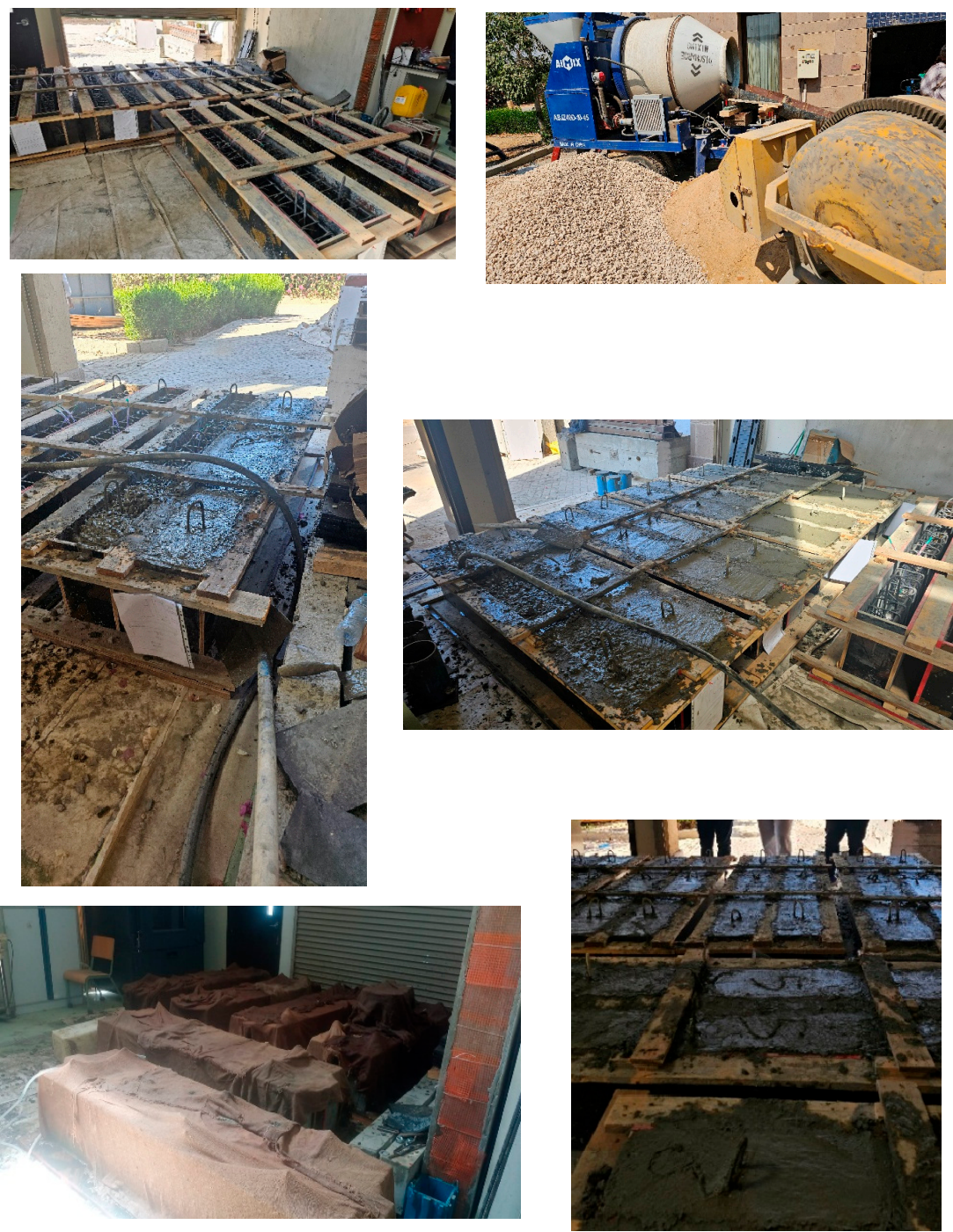
Figure 2. Casting and curing the beams.
