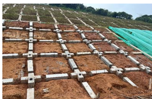
Figure 10. On-site assembly diagram of prefabricated longitudinal and transverse beams with cross nodes.
