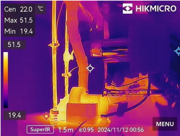
Figure 3. - Thermal Analysis of Steel and PVC Pipes Near Ductwork.
