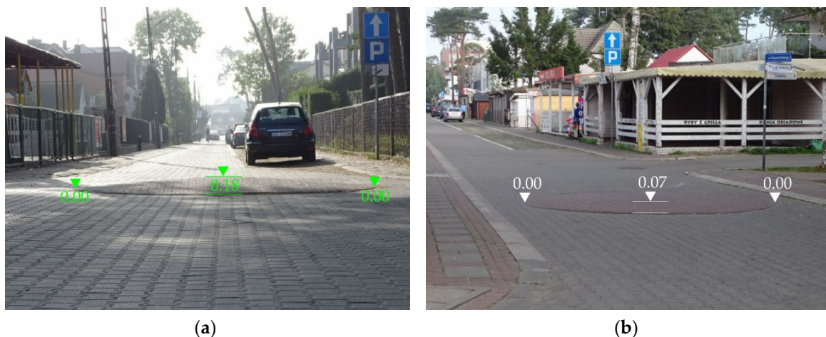
Figure 9. Analysed traffic circles: (a) No. 3 – \Delta h = 0.17 m; (b) No. 6 – \Delta h = 0.08 m (all dimensions in metres). Source: photo by Alicja Sołowczuk.
