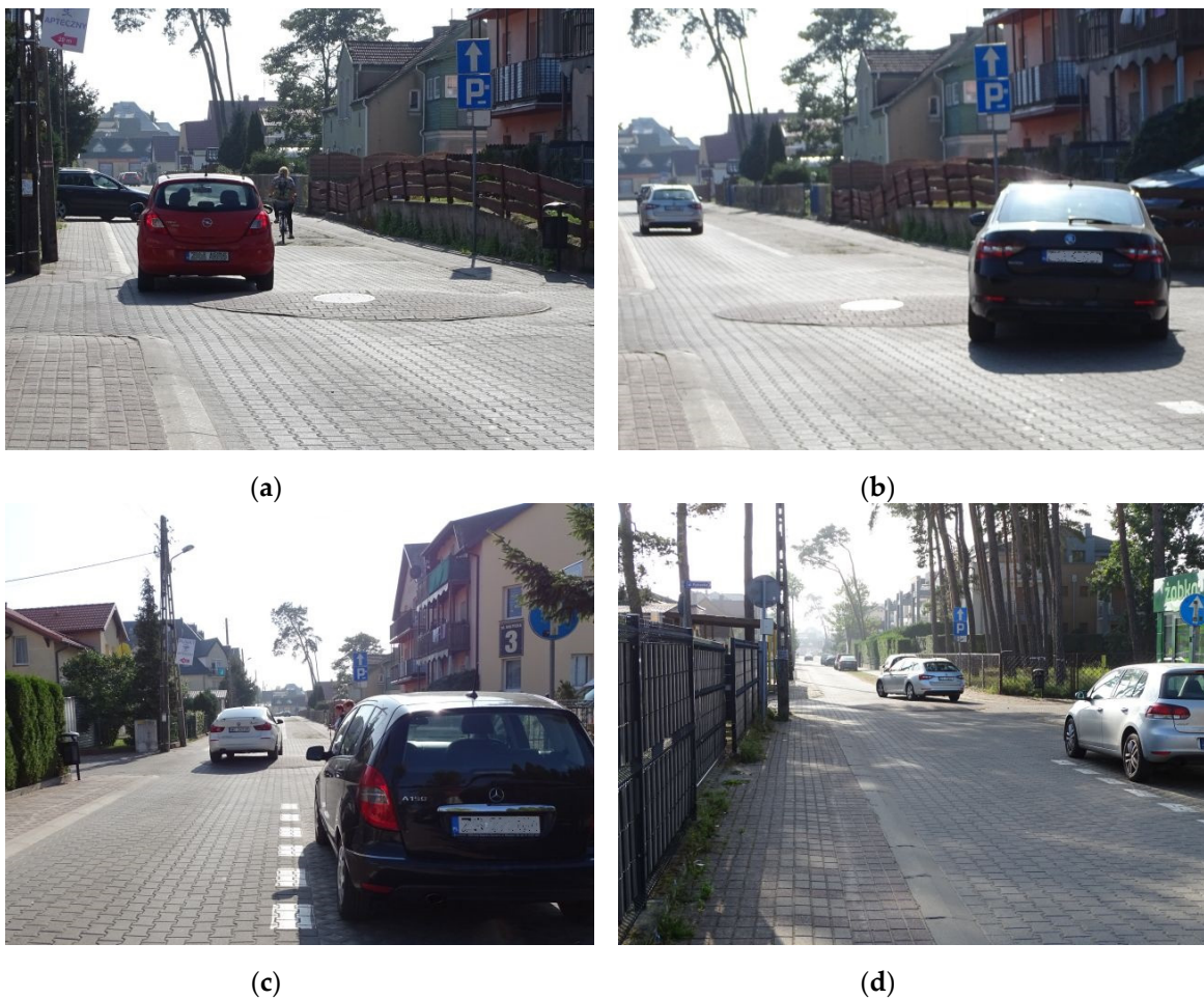
Figure 14. Examples of passenger cars driving through traffic circles: (a) traversing the island on the left-hand side; (b) traversing the island on the right-hand side; (c) traversing through the central part of the island; (d) bypassing the island by pulling right. Source: photo by Alicja Sołowczuk.
