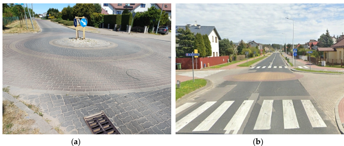
Figure 2. Examples of traffic circles used in Poland on two-way streets: (a) an example of a sectioned-off central island on a raised junction in Mierzyn, including traffic signs directing the traffic around the island. Source: photo by Alicja Sołowczuk; (b) example of coloured/textured surface used on the central island of a raised junction in Puławy. Source: Google Earth [5].
