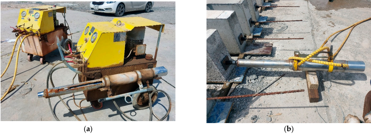
Figure 8. (a) Post-tensioning machine. (b) tendon jacking.
