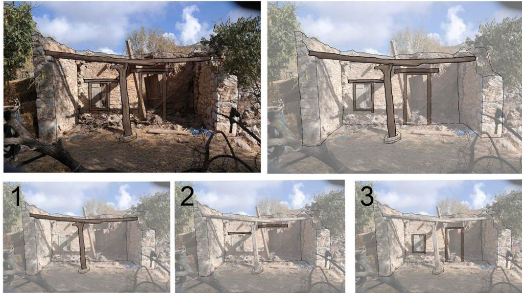
Figure 15. Wooden elements on a house in Taşlıca. (1) structural elements (2) hatul for openings. (3) opening frames.
