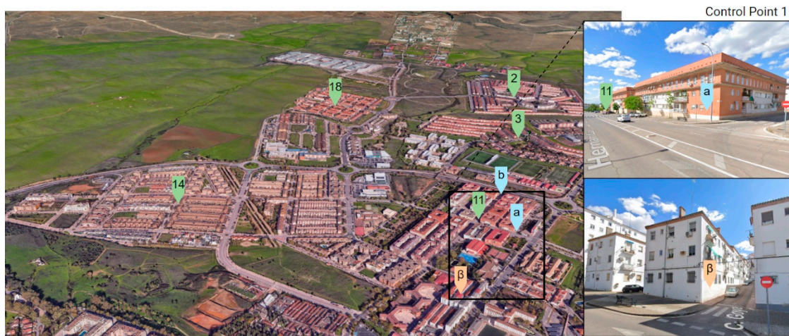
Figure C1. Control point CP1 in the North zone.
