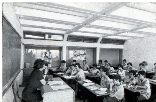
Figure 12. Ram Karmi, Lady Davis school: classroom with the waffle slabs, photographer unknown, 1973.
