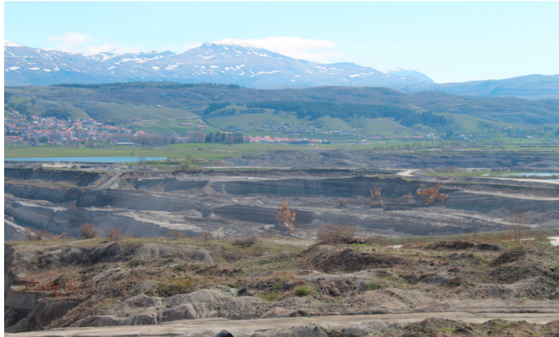
Figure 1. Gacko open pit (photographed by the author of the article: N.S.).
