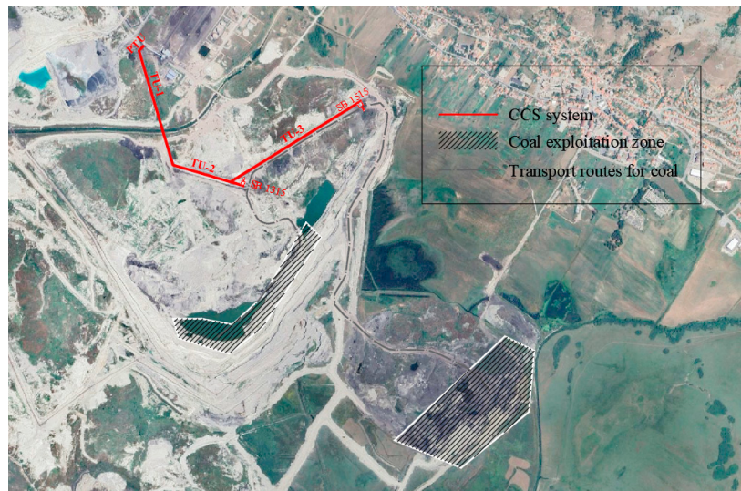
Figure 2. View of the CCS system (Source Google Earth).
