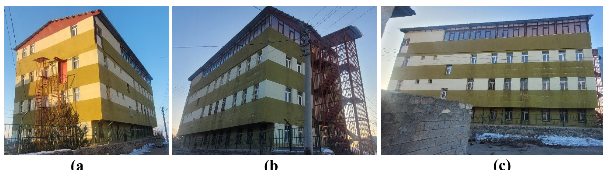
Figure 2. Various views of the examined educational building: (a) Southeast facade; (b) Northeast facade; (c) east facade.
