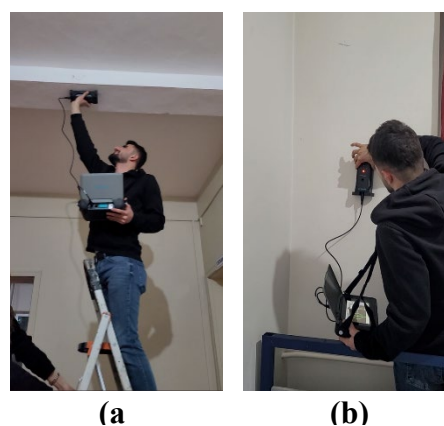
Figure 8. Images from the reinforcement scanning process: (a) Beam; (b) Column.
