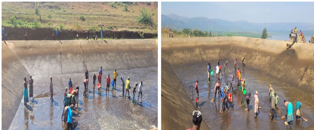
Figure 7. Desilting storage reservoir at Nasho GFI scheme.
