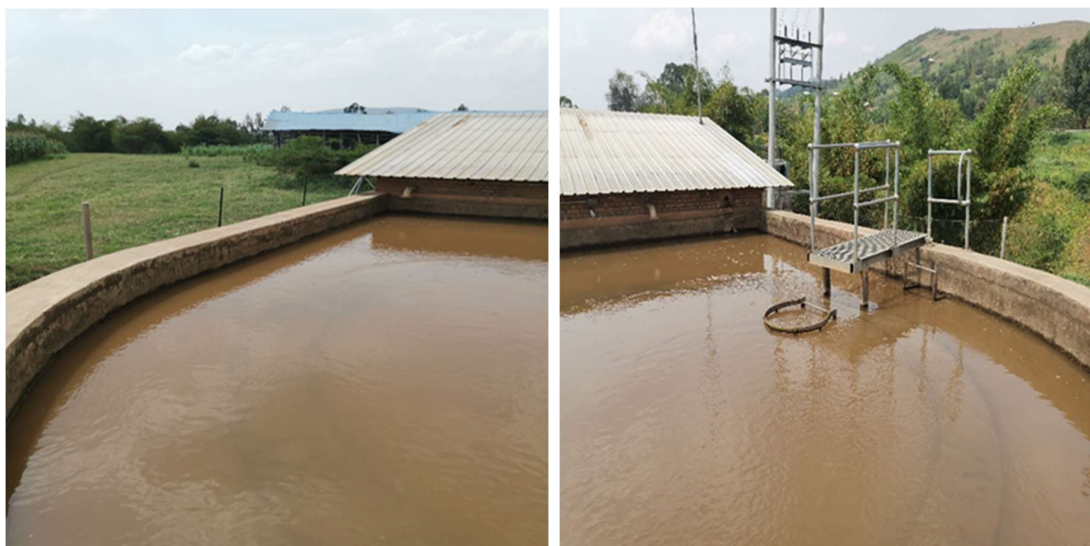
Figure 9. Storage reservoir at Kagitumba irrigation scheme.
