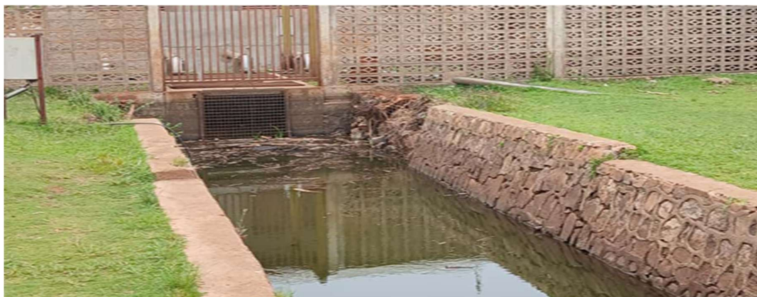
Figure 3. Conveyance canal at Nasho GFI scheme.
