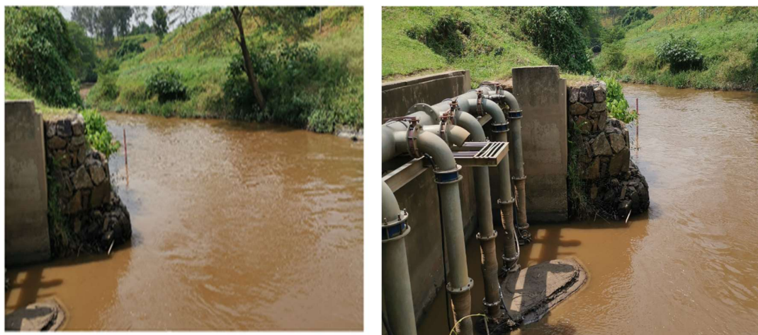
Figure 10. Intake structures at Kagitumba irrigation scheme.
