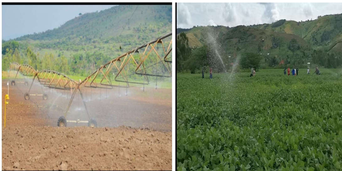
Figure 11. Irrigation system at Kagitumba irrigation scheme.
