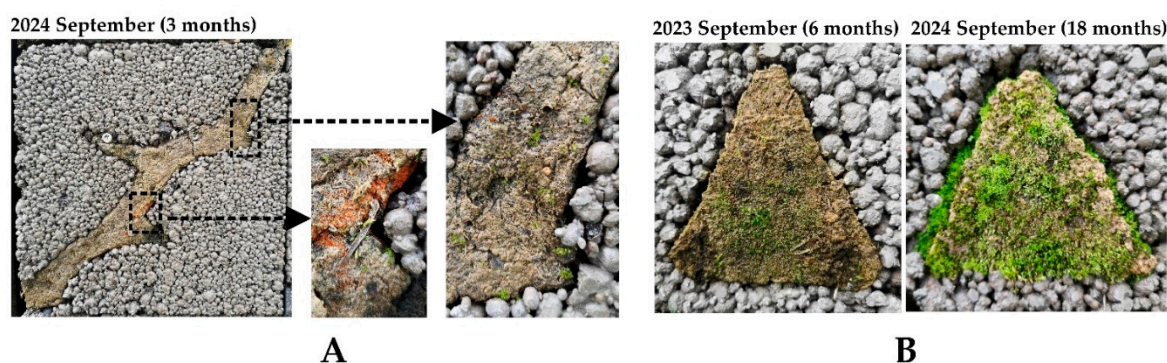
Figure 5. Biological growth on the LLC: after three months of field exposure the initial growth of fungi and mosses start to be visible on panels of test Series 3 (A) and growth evolution in 6 – 18 months period on panels of test Series 2 (B).
