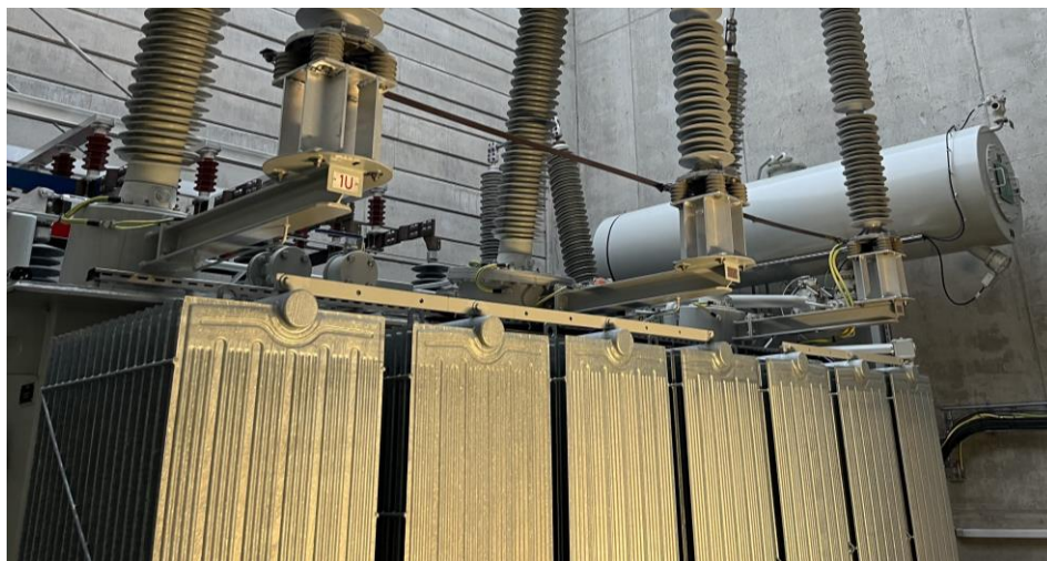
Figure 1. The three-phase 40 MVA power transformer in operation in the substation. The photo focuses on the auxiliary equipment: the radiators in the front, the HV-bushings and the surge arresters on the top, and the oil expansion tank in the back.
