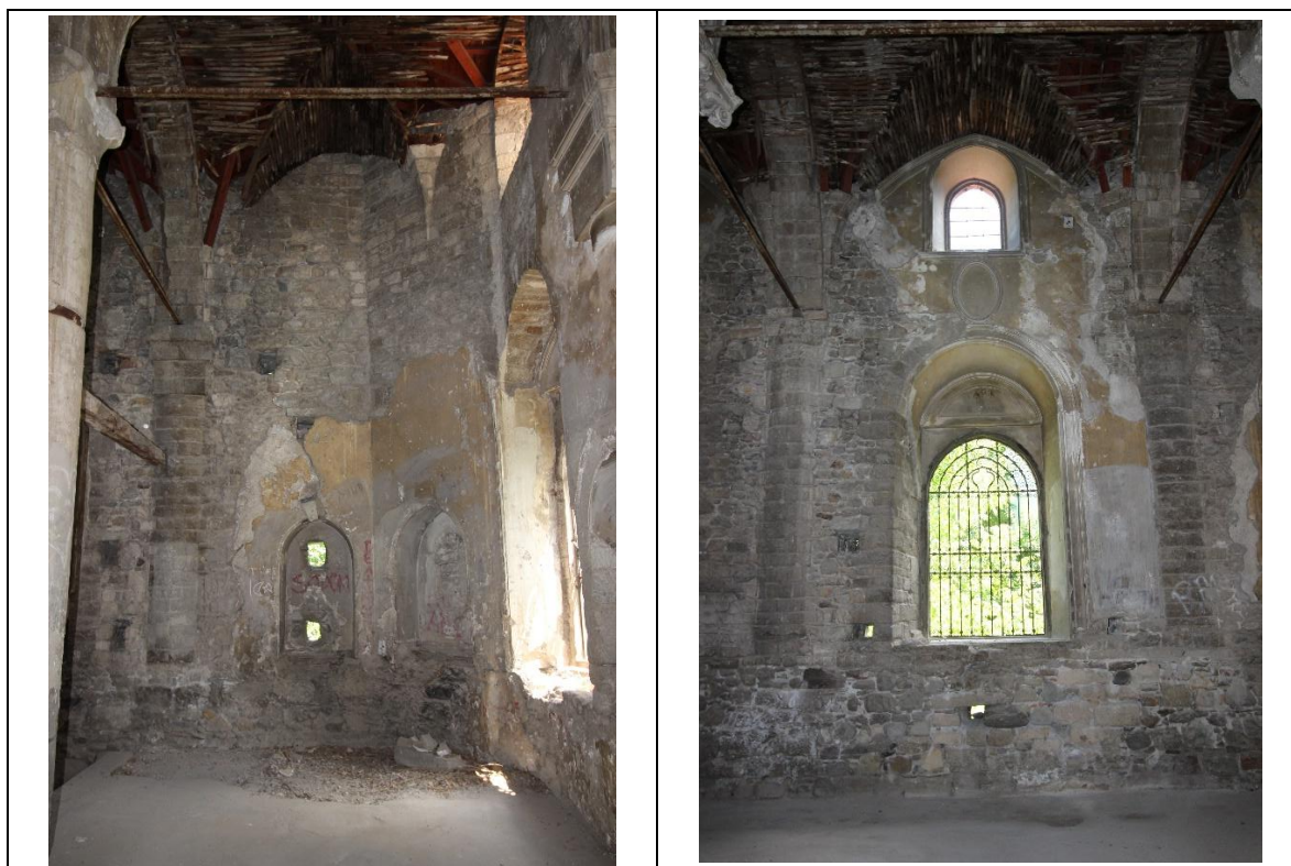
Figure 7. Wall Bonding Technique in the Naos (Author's Personal Archive).
