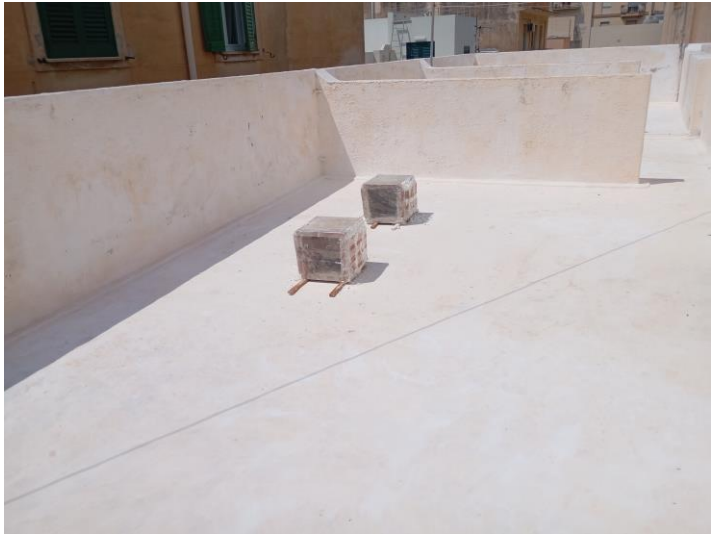
Figure 3. The prototypes placed on the roof.
