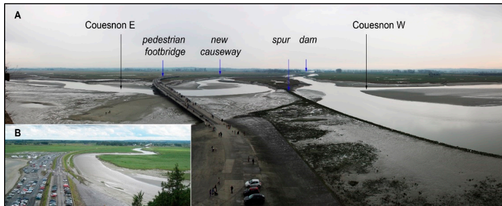
Figure 11. Photographs taken from the ramparts of the Mont-Saint-Michel (southward views). A. 21 February 2023. B. 31 May 2007. Cars were parked very close to the Mont in 2007. In the background, demolition work of the Caserne dam has begun (a construction crane is visible). The Couesnon river is largely meandering in the schorre and located only to the west of the causeway. The new facilities separate the Couesnon river in different parts (Couesnon east and west, channel along the spur) in 2023. The schorre has been partly eroded (see text for details).
