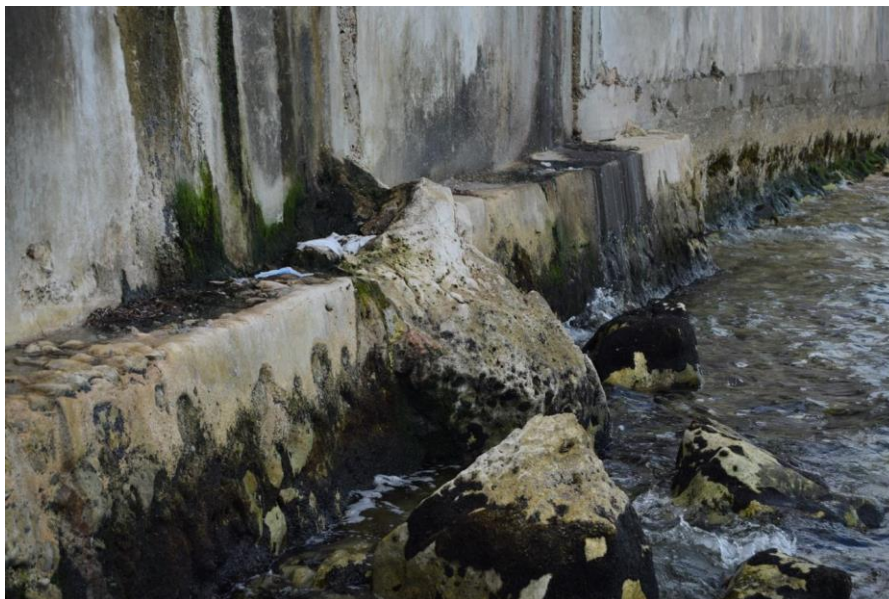
Figure 2. Intertidal concrete structures such as the base of this fisherman's house, built over a rocky shore, exhibit a heterogeneous coverage of microorganisms. Lerma village, Campeche, Mexico.
