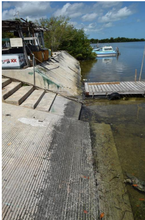
Figure 1. Concrete docks for artisanal fishing boats in Campeche, southern Mexico. Note that areas reached only by the marine spray appear devoid of (visible) microbial colonization, whereas intermittently submerged surfaces are covered by black biofilms. Permanently submerged areas are heavily covered by phototrophic communities. San Francisco de Campeche, Campeche, Mexico.
