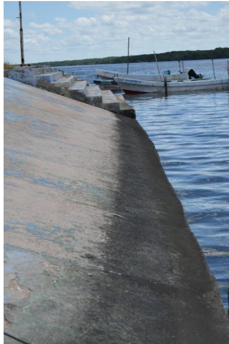
Figure 3. Biofilms covering concrete surfaces often exhibit a black phenotype indicating the likely presence of scytonemin-producing cyanobacteria as a functional adaptation for water stress and excessive insolation. San Francisco de Campeche city, Campeche, Mexico. .
