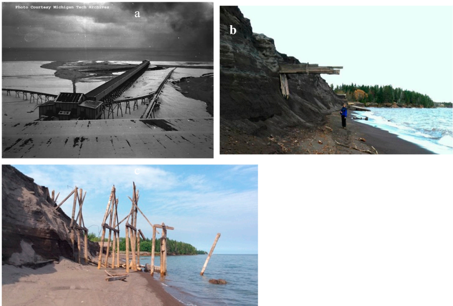
Figure 2. Gay Stamp Sand Pile. A) primary wooden discharge launder distributing tailings onto the Gay Pile, around 1922, with smaller sluices conveying stamp sand and slime clays laterally (courtesy MTU Archives). B) Photo of 6-8m high stamp sand bluffs on July 2008 off Gay, showing a buried small lateral sluiceway protruding out of the pile along the shoreline. Lake Superior waters are to the right; the dark beach sands are stamp sands with intermixed slime clay layers. C) Bluff photo from about the same location in 2019, when shoreline erosion (ca. 7-8m/year) reached the buried primary launder support beams, just before bluff removal. (B & C photos, W.C. Kerfoot).
