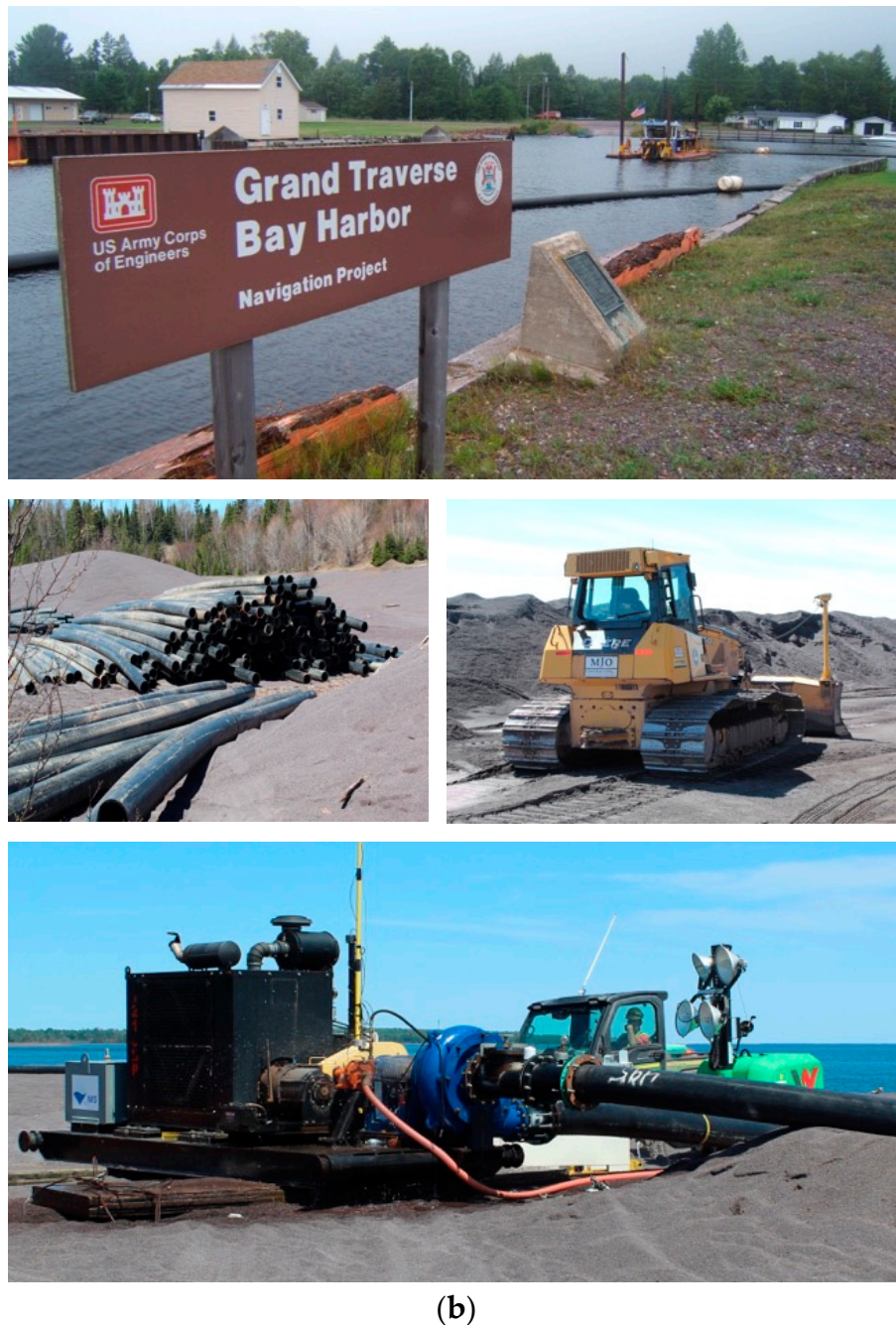
Figure 13. (a). Army Corps initial remediation plans and implementation steps (dredging & berm placement): a) Dredging and excavation of stamp sand from the Traverse River Harbor (2017-21) and “Trough” (2020-21) followed by deposition into the “Berm Complex”. Removal of stamp sand north of the Seawall (orange site) was later enlarged from 50’ to around 500’. (b). Initial dredging begins at the Traverse River Harbor (top, fall of 2017); 5-7 km of plastic pipes (middle) and pumping stations (bottom) used to transport stamp sand from the Traverse Harbor and “Trough” to the “Berm Complex” (2019-2021). Shovel (middle right) used during berm wall construction. (map courtesy U.S. Army Corps, Detroit; photos W.C. Kerfoot).
