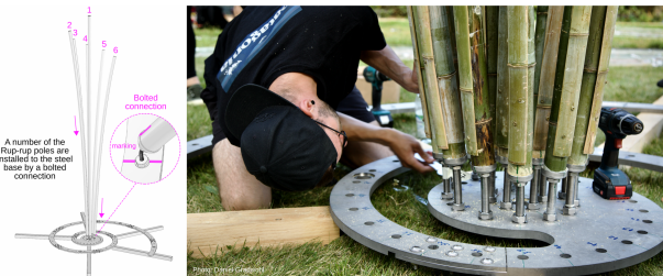
Figure 23. Installing the primary structure
