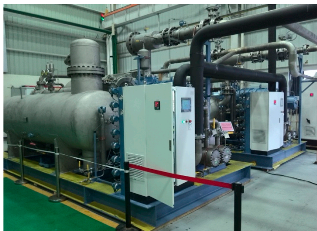
Figure 6. Large-scale screw helium compressor units used in the refrigerator (2500 W@4.5 K/500 W@2 K).
