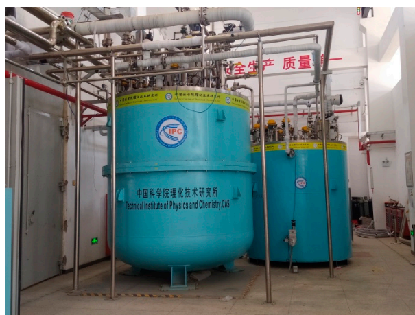
Figure 7. Large-scale cryogenic refrigeration cold boxes for liquid helium to superfluid helium temperature range (2500 W@4.5 K/500 W@2 K).
