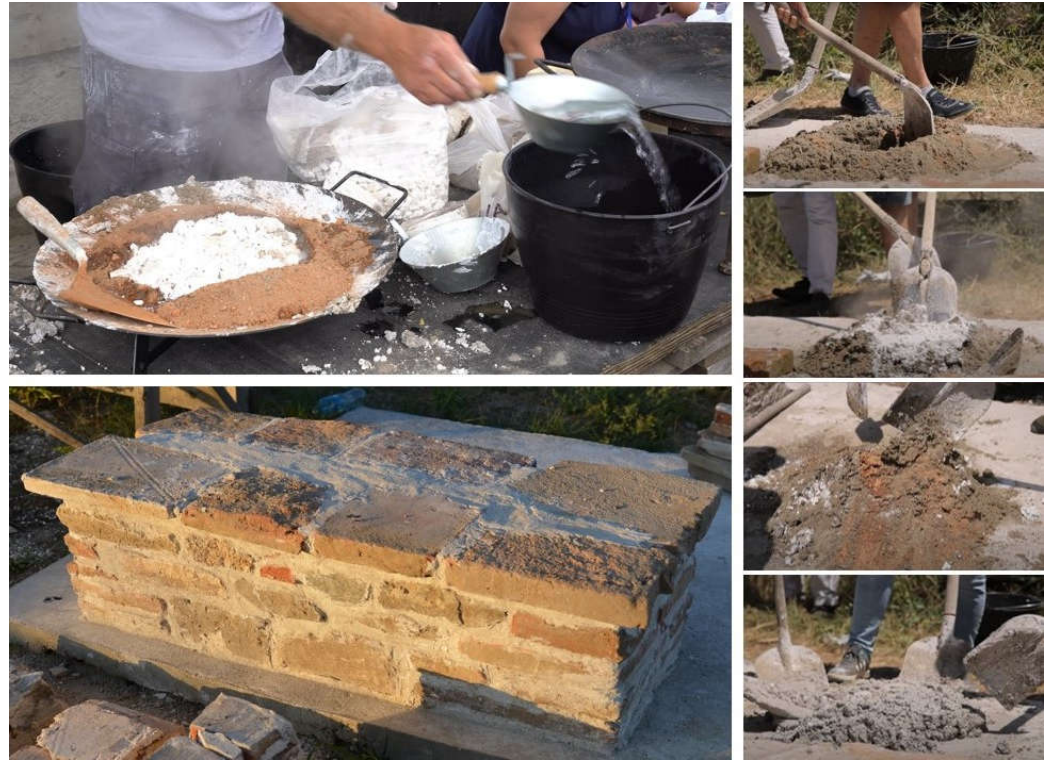
Figure 11. Hot mixing during the MoDeCo2000 workshop and building a wall structure with lime mortars having natural brick addition. Photo-documentation of the MoDeCo2000 project.
