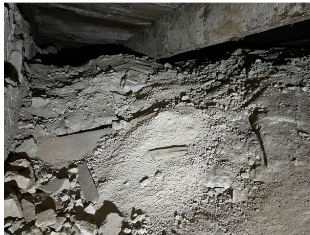
Figure 17. Back of the vault of the Mas Palace. Source: Authors.
