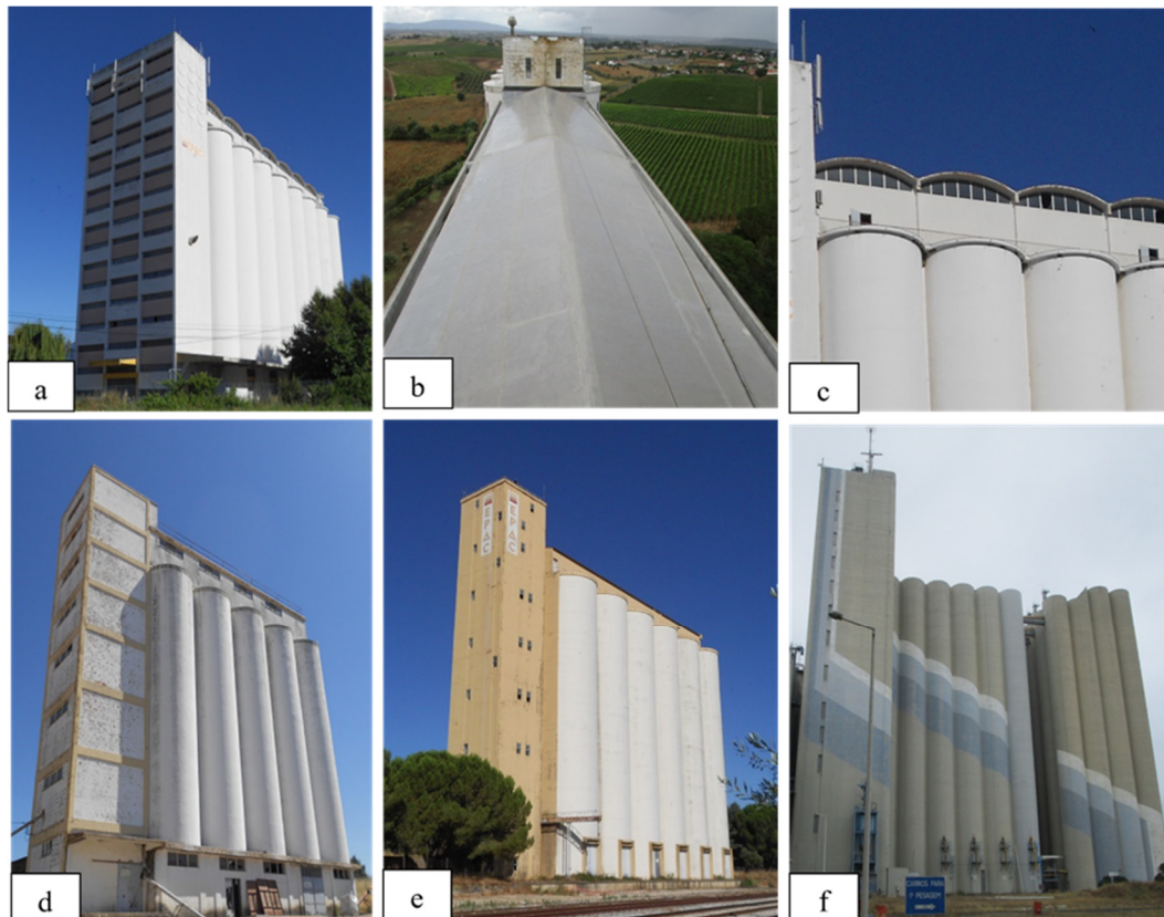
Figure 5. EPAC silo construction details: a) tower at the silo in Evora, Alentejo, b) gable roof on the silo in Vale Figueria, Centre, c) curved roof on the silo in Evora, Alentejo; Different types of
