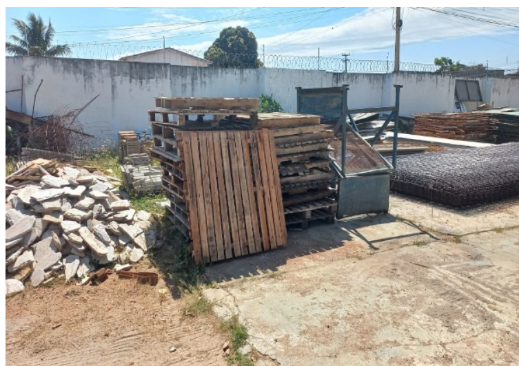
Figure 3. Open-air storage of hardware, timber and stones for reuse by construction companies in Mossoró/RN. Source: Author, 2024.
